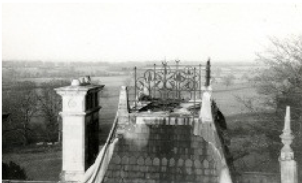
View to north of Tilgate House from roof, c1960
