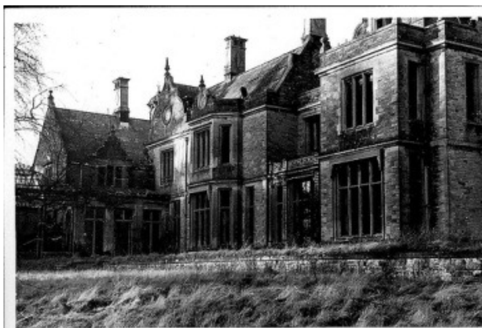
Tilgate House, showing low wall around building (extant), c1960
