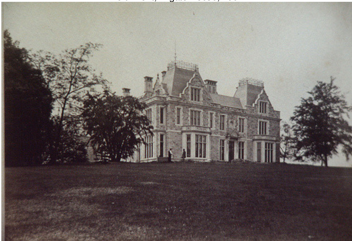
East front, Tilgate House, c1910
